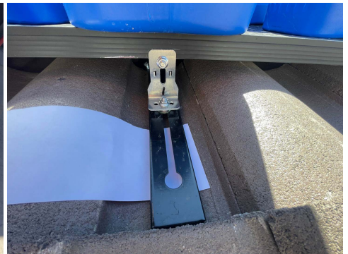
PHOTO 6: Load 2 - Bracket under load
