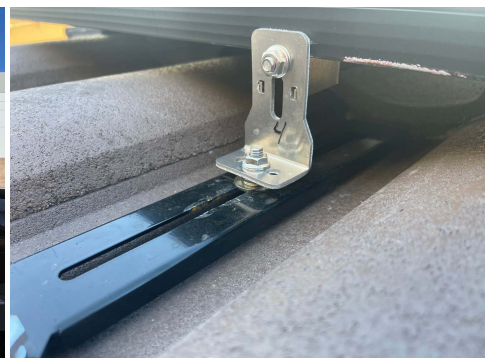
PHOTO 9: Unloaded Bracket - after tests
