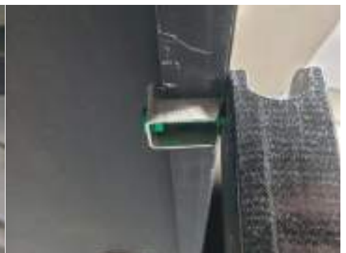
Figure 18: IR Ballast frame connection to solar panel
