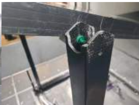
Figure 17: IR Ballast frame connection to solar panel
